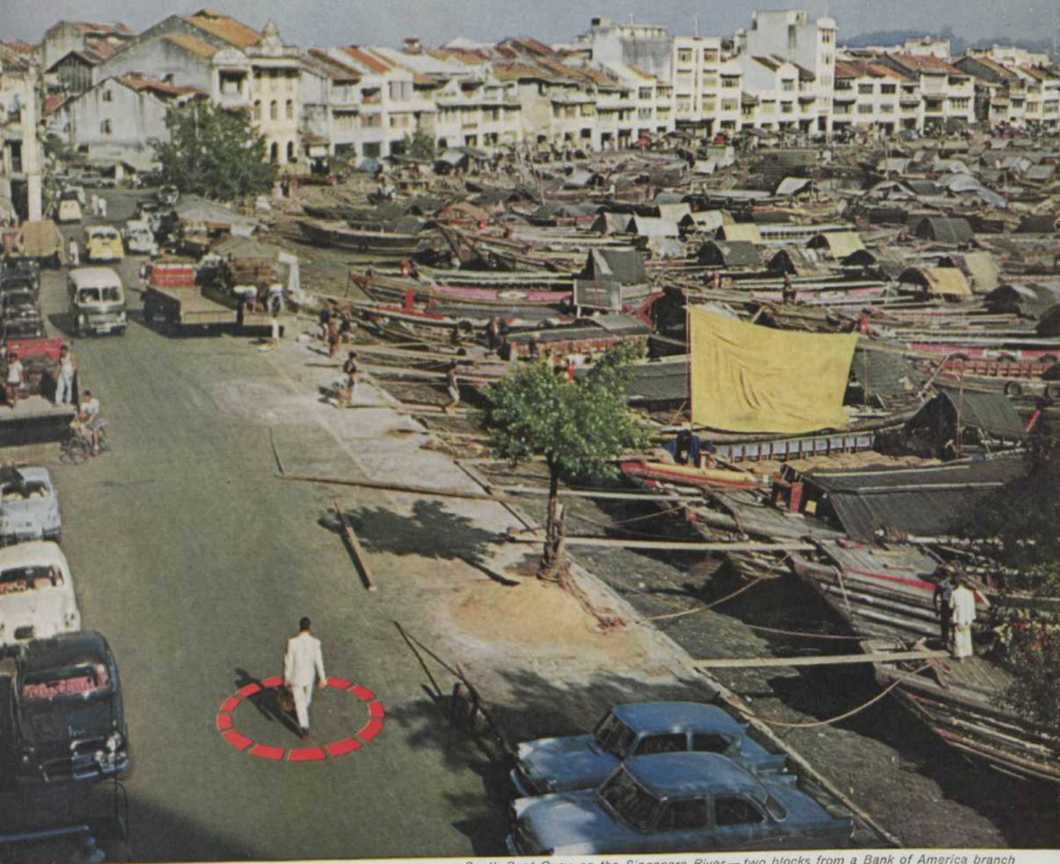
South Boat Quay, on the Singapore River—two blocks from a Bank of America branch
